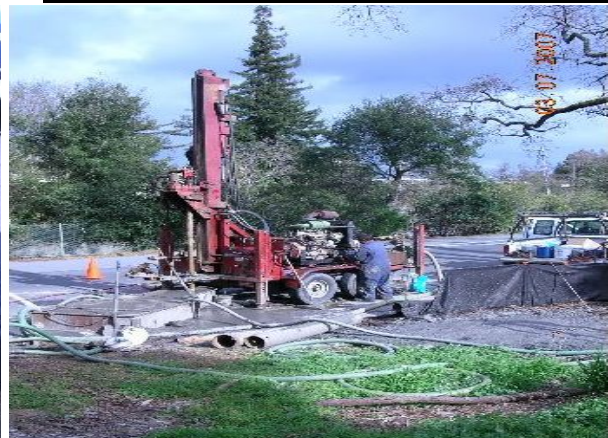
Drill Rig for Geothermal Test Bore
