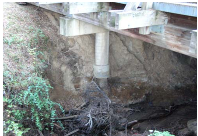
Creek at bridge between parking lots 1 and 2
