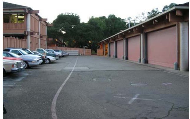
Looking west at Pomo 2 and work yard
