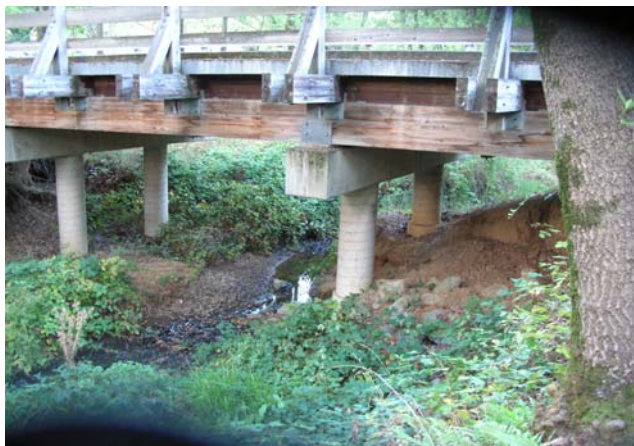
Creek at bridge between parking lots 5 and 6
